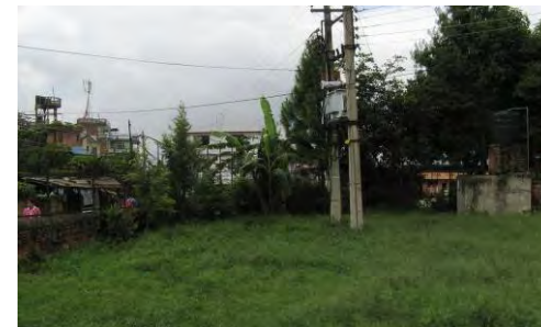
Sector: electricity poles
